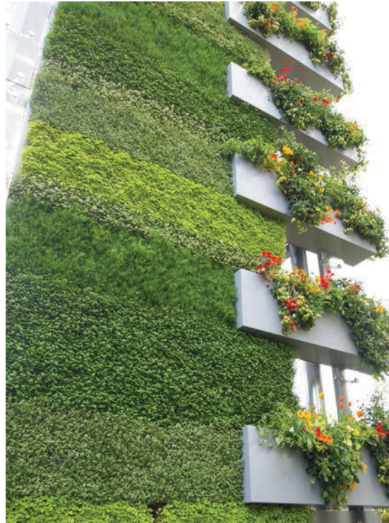
Picture 10.1 Living wall & planted balconies
