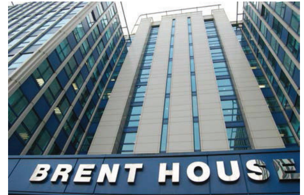
Picture 5.3 Brent House, Wembley High Road
