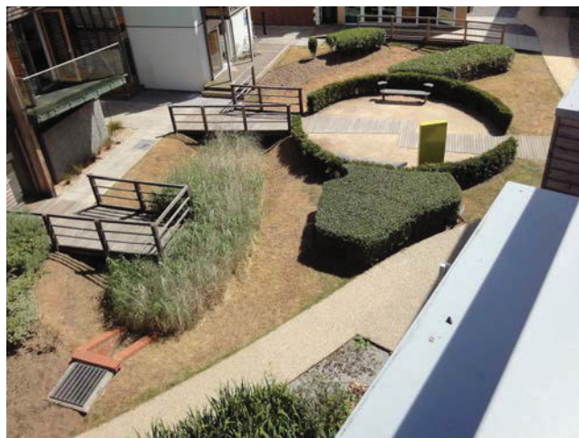
Picture 10.2 Sustainable urban drainage scheme
