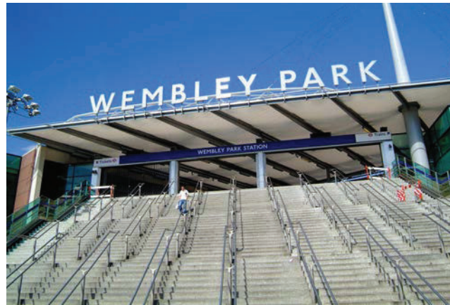
Picture 4.21 Wembley Park Station
